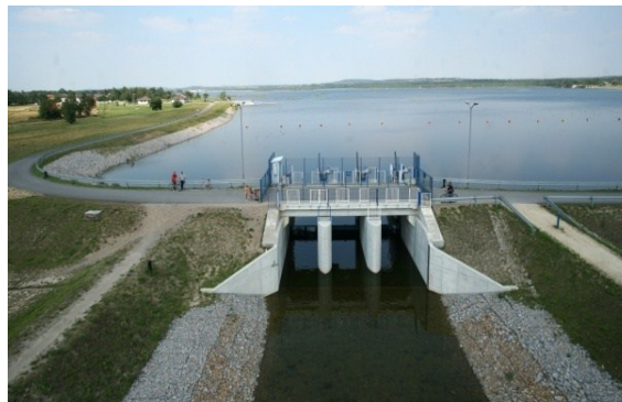
The Kuźnica Warężyńska flood control reservoir
