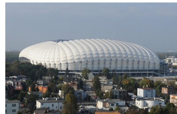
Football stadium in Poznań
