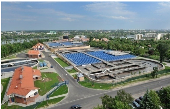
The Left-Bank Wastewater Treatment Plant in Poznań
